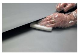
The membrane should then be washed with a suitable cleaning detergent mixed with warm water. The area should be scrubbed and rinsed down to ensure all contaminants are cleared from the area.
